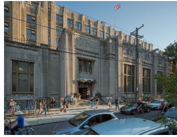
Figure 25. Image of Bok Building (Source: Bok Website)
