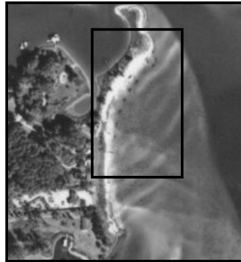
Figure MOB3.1. Aerial photo of the breakwater at Mobjack Bay 3, VA.
