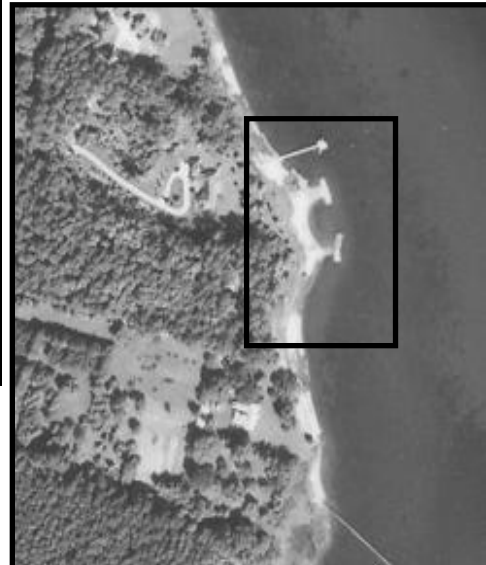
Figure MOB7.1. Aerial photo of the breakwater at Mobjack Bay7, VA
