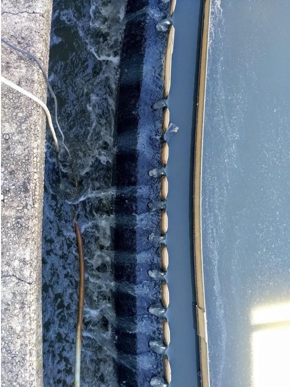
Figure s4: Source primary effluent for pilot MFC system, submersible pump in primary effluent channel of a west primary clarifier, DC Water Blue Plains, Nov 29 2018
