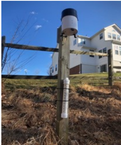
Figure A.5: A tippet bucket rain gauge and atmospheric pressure transducer, placed within a protective PVC housing, mounted to a fence post within an open field approximately 100 yards from the outfall of terminal dry detention Pond 6.
