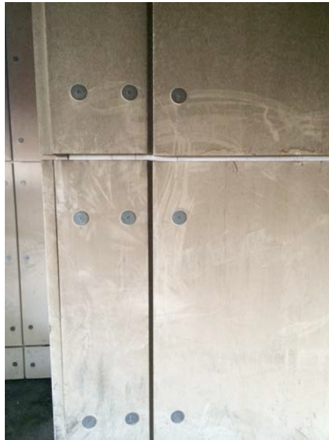
Figure A.1: New Padgenite Insulating Panels on First Floor
