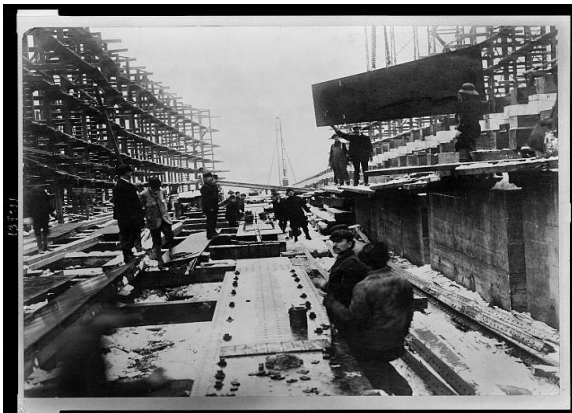
Image 29: Laying the Keel of the North Dakota at Fore River Yards, First of the Amer. Dreadnoughts—20,000 tons. 1907. Bain Collection. LOC Prints and Photographs Division.
