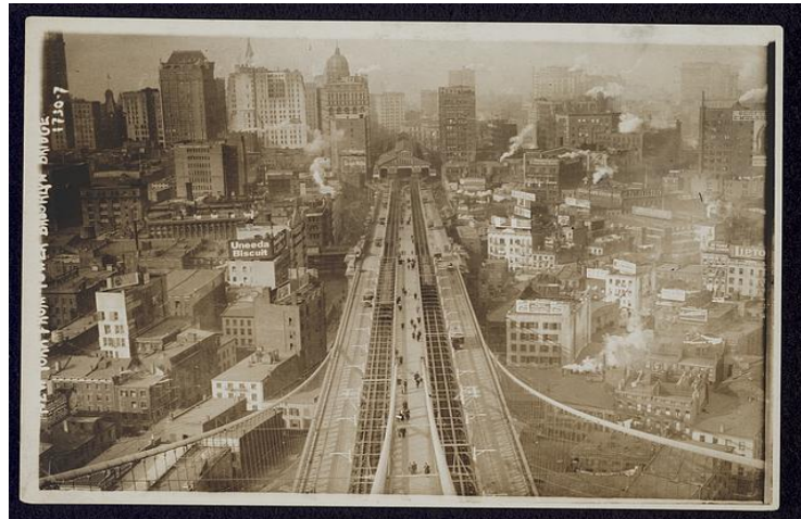
Image 14: New York from Tower of Brooklyn Bridge. Bain News Service. Between 1907 and 1915. Bain Collection, LOC Prints and Photographs Division.
