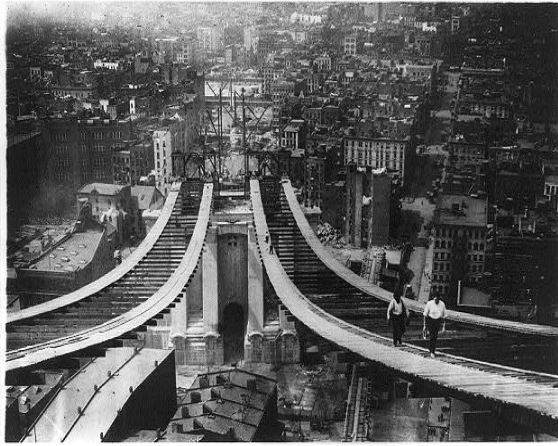
Image 25: Footpaths of Manhattan Bridge [when the bridge was being built]. Bain News Service. Between ca. 1907 and ca. 1915. Bain Collection. LOC Prints and Photographs Division.
