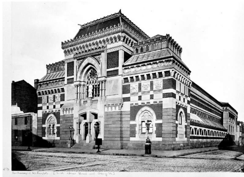
3.7. Frank Furness, architect, Pennsylvania Academy of Fine Arts (Broad and Cherry Streets., S.W. corner), photograph by Robert Newell, Library Company of Philadelphia, ca. 1875, P.9062.21b (Brenner), 7 ½ x 9 ½ inches, http:// www.brynmawr.edu/iconog/nwl/Newell.html , accessed 3/23/06.
