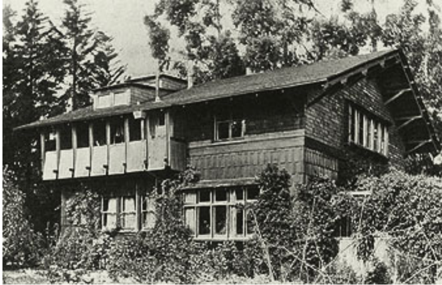
4.26. Bernard Maybeck Home , Berkeley, California, as seen in 1902 from rear, Dimitri Shipounoff collection, BAHA archives, http://berkeleyheritage.com/berkeley_landmarks/maybeck_on_grove.html , accessed 4/17/07.
