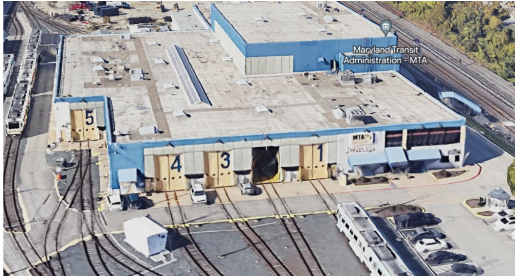
Figure 13: North Avenue overhead garage doors on the front of the facility.
