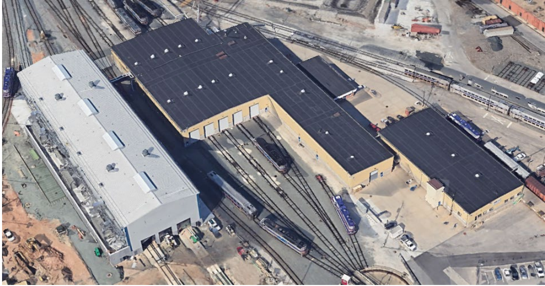
Figure 16: Overhead garage doors at the Riverside MARC Facility
