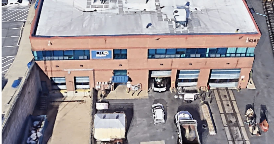
Figure 15: Overhead garage doors present at Old Court Facility
