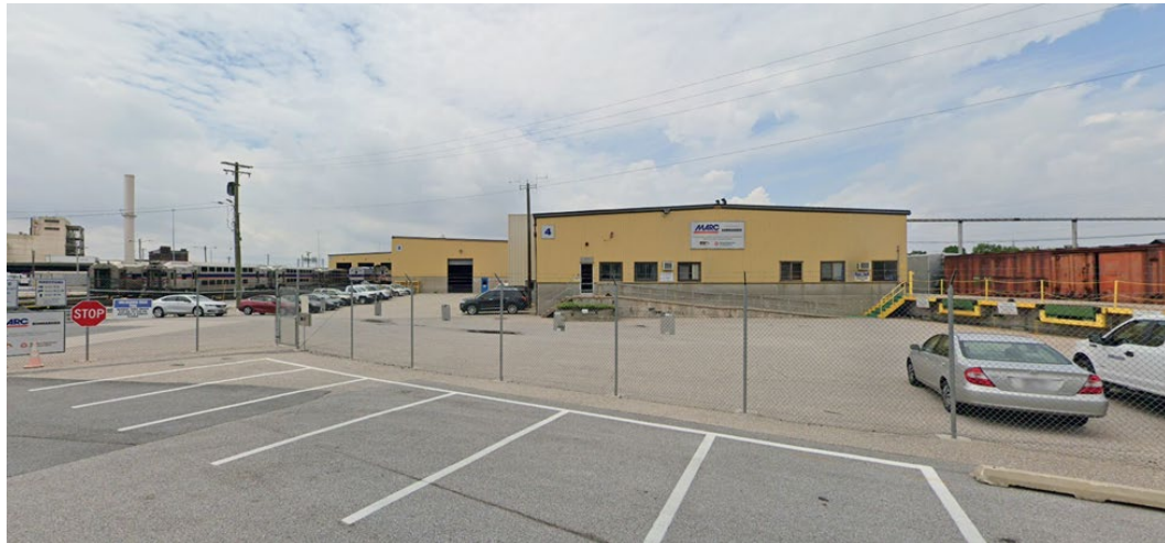
Figure 8: Street view of MARC Riverside Maintenance Facility
