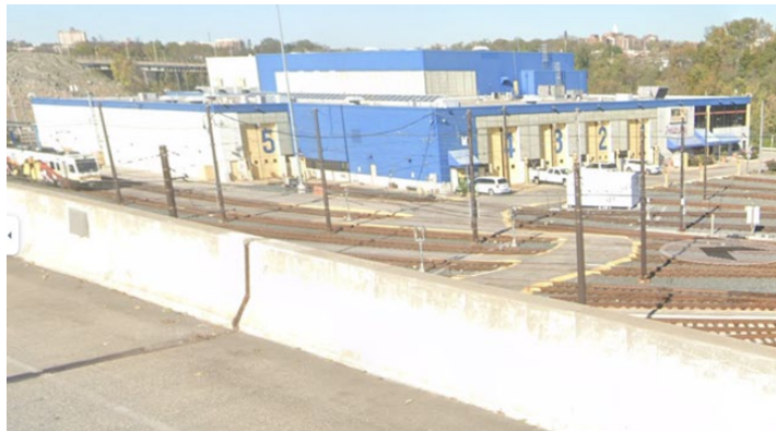
Figure 3: The street view of the North Avenue Light Rail Maintenance Facility.
