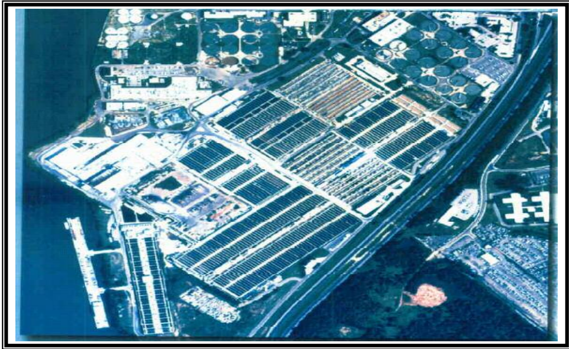
Appendix IV - 1: An Aerial view of the DC WASA blue plains AWWTP
