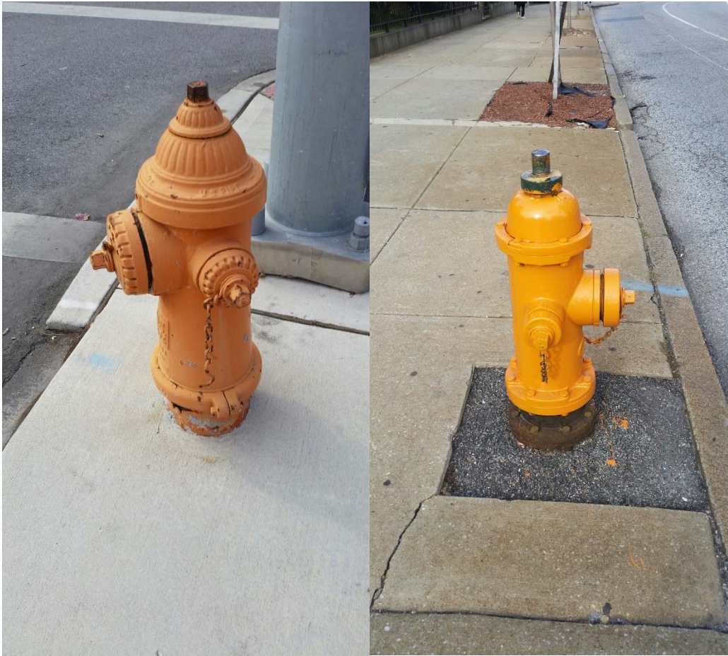
Figure 5-10. Old and New Fire Hydrants
