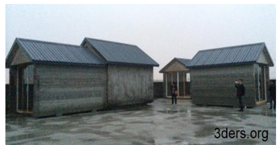
Figure 30. 3D printed houses constructed in one day (“China's WinSun Unveils Two New 3D Printed Buildings” 2015, January 28).
