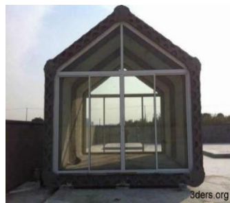
Figure 30. 3D printed houses constructed in one day (“China's WinSun Unveils Two New 3D Printed Buildings” 2015, January 28).
