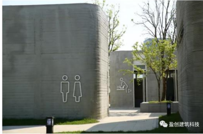
Figure 31. Winsun's 3D printed toilet in Suzhou Yangshan in Jiangsu (Winsun's Website, n.d.).
