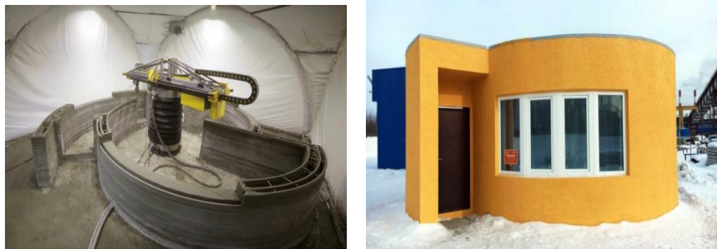
Figure 6. Apis Cor's 3D printed building ("Thanks to 3D printing, you can now build a home in just 24 hours", 2018, February 09).
