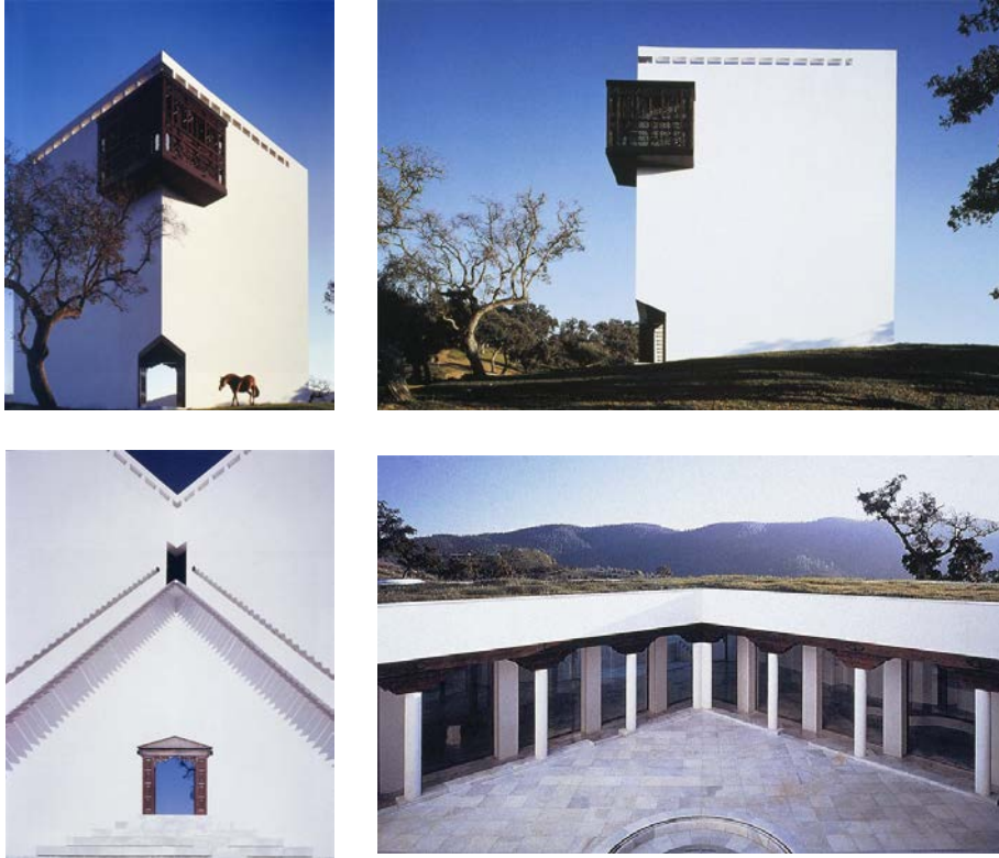
Figure 6 – Photographs of Casa de Retiro Espiritual
