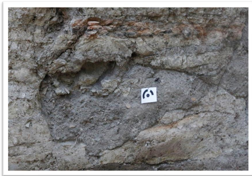
Figure 4. An example of the type of coded marker utilized as a GCP on the Western wall of Block 4 (photograph by the author).
