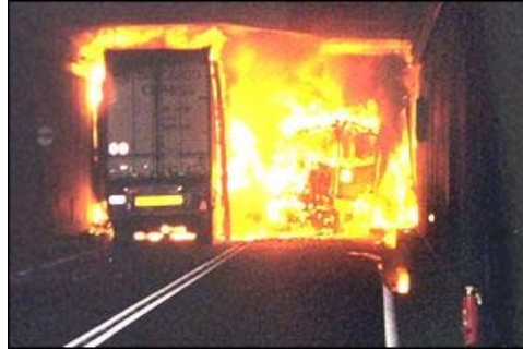
Figure 1. Photo showing a tunnel involved in a fire ( www.etnfit.net )
