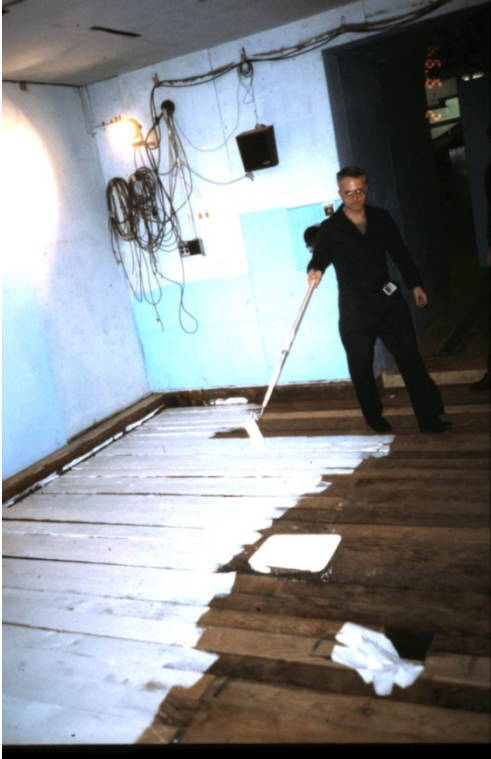
Figure 9. Application of gadolinium paint in exposure room 2. Although the literature describes a controlled application, this photo would tend to indicate that control measures were less thorough than described. AFRI photo.
