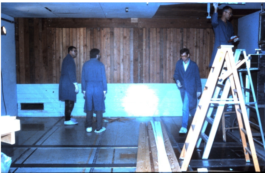
Figure 8. Installing the Masonite lining in exposure room 1. AFRRRI photo.
