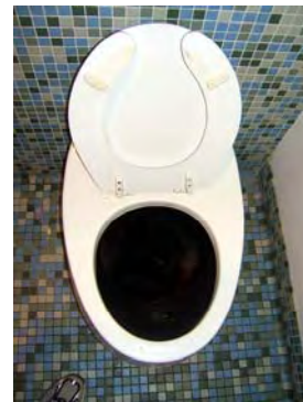
Compost Toilet at Chesapeake Bay Foundation
