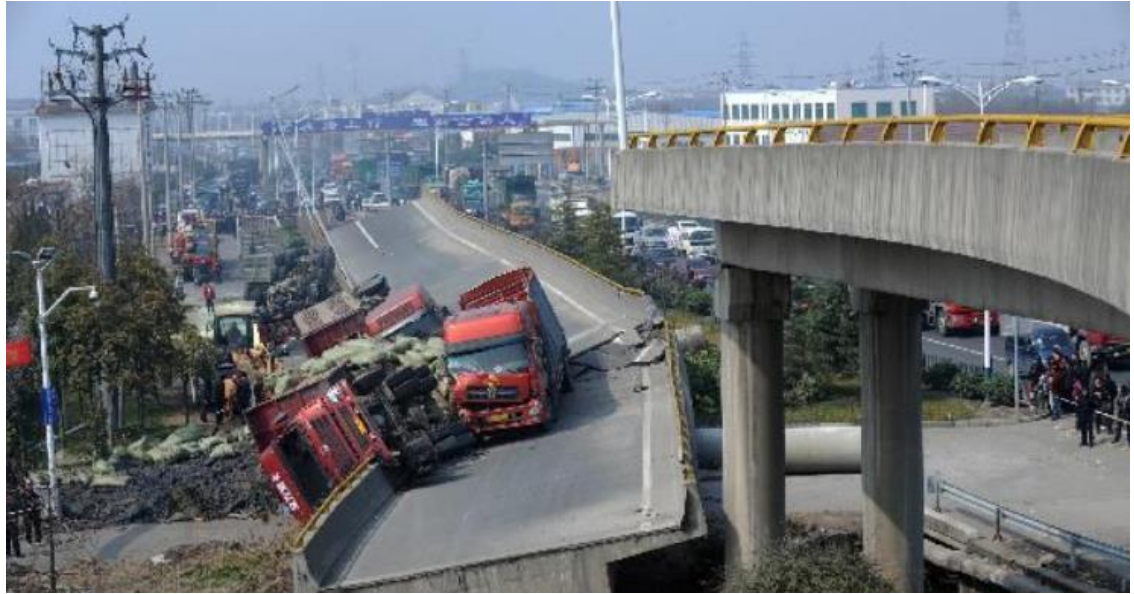
Figure 1-1 Shangyu curved bridge accident
