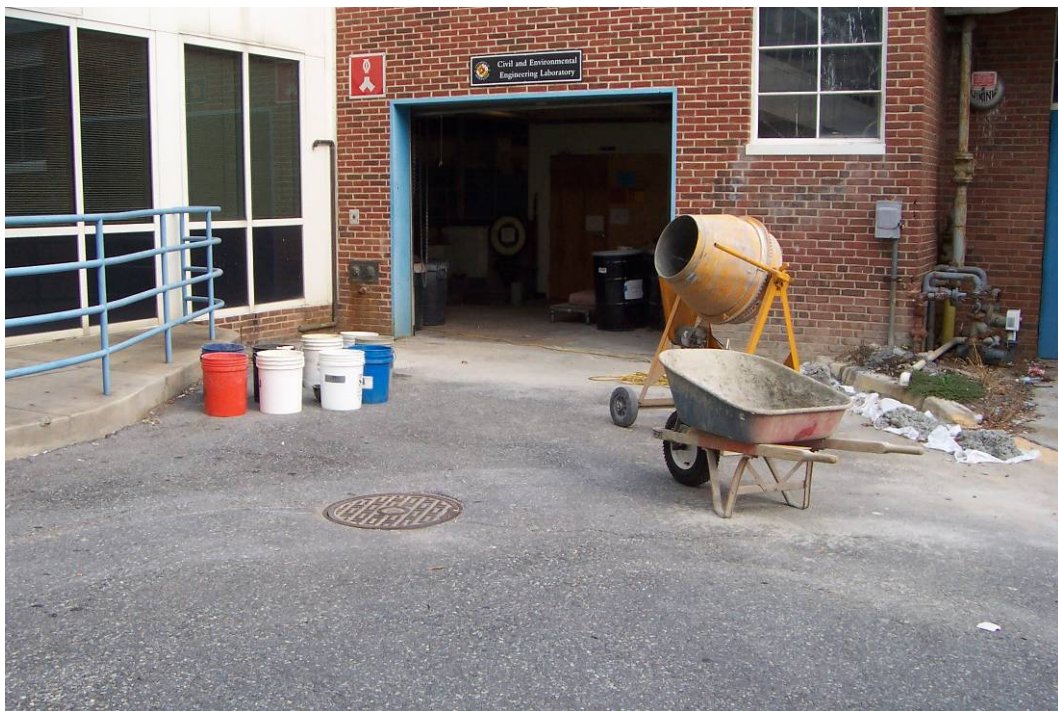
Figure 5.11 - Concrete Mixer with Wheel Barrel at UMD Structural Lab
