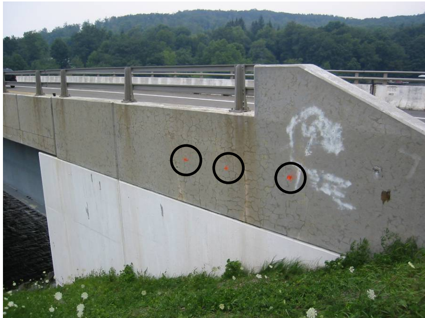
Figure 2.2 - Coring Locations on Bridge No. 1102100 ( U.S. 219 over Deep Creek Lake) (Amde et al. 2004a)
