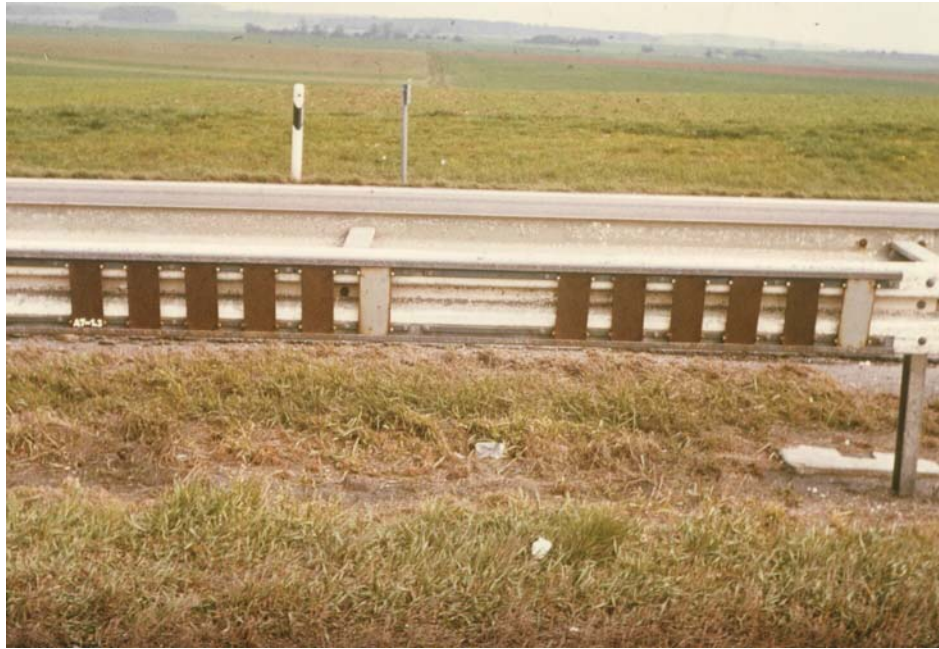
FIG. 8.7(a). Highway site in Merklingen (Hein 1981)
