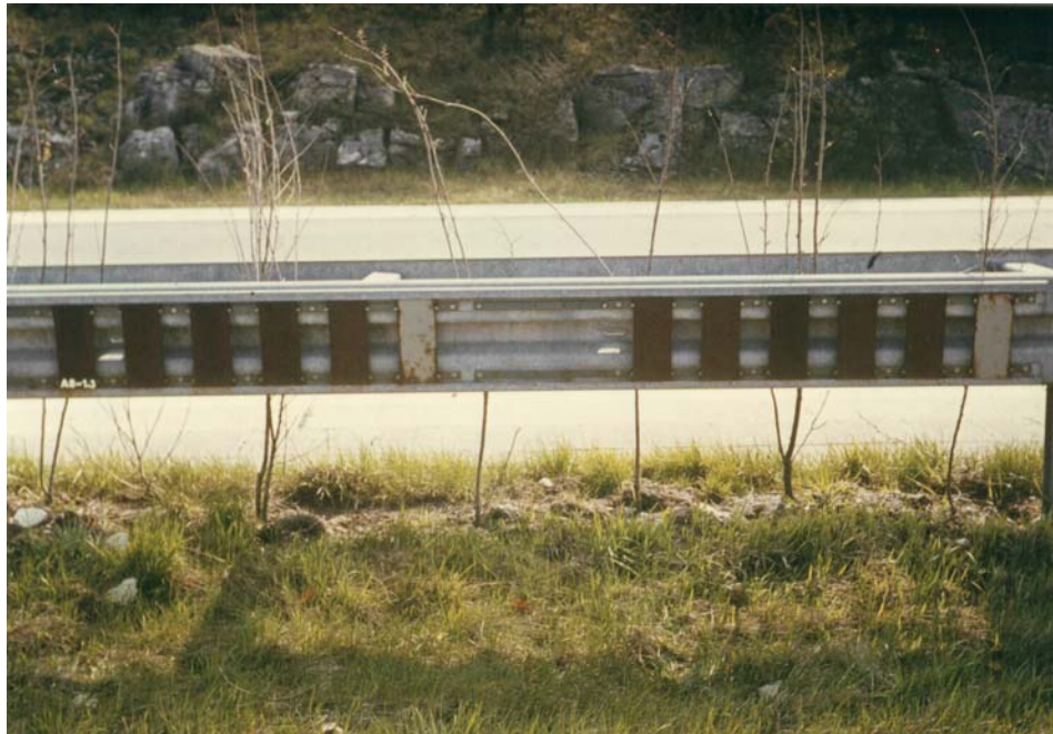
FIG. 8.8(a). Highway site in Trockau (Hein 1981)
